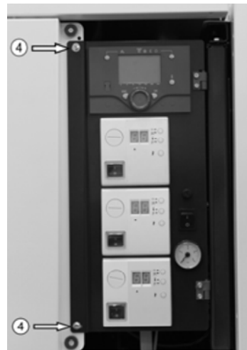
4. Using a 4mm Allen Key loosen the two captive bolts.
